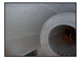
The **RESCOBOND** product range includes the world renowned AA-22S. Since it was first developed and Patented in 1956, it has been the Petrochemical Industries standard in erosion resistant castables for cyclone, and other highly erosive areas.
