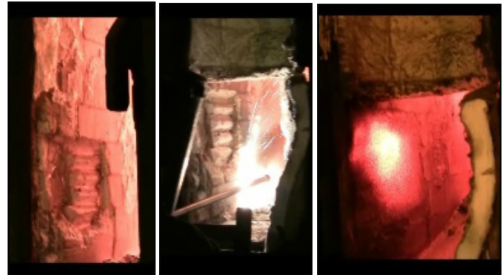
From left to right: damaged wall prior to repair, welding in progress, finished repair.
